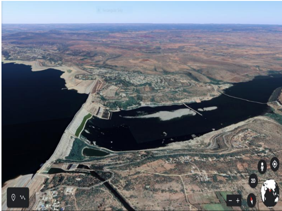
Fig 2: Satellite image of Nagarjuna Sagar Dam
